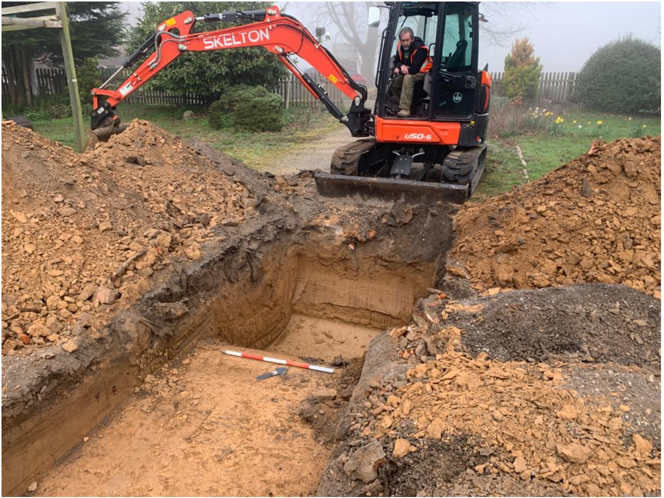
Plate 12. Working shot of excavation of test pit in Trench 1.
